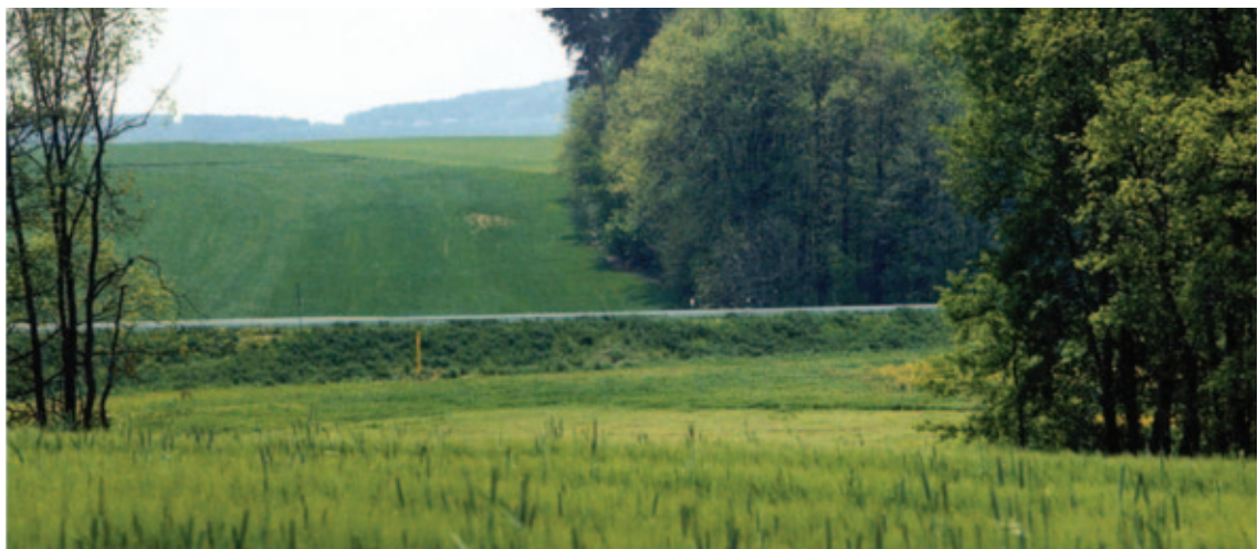
Figure 6: Reinstating the environment – minimal visual impact of pipeline (Source E.ON)
